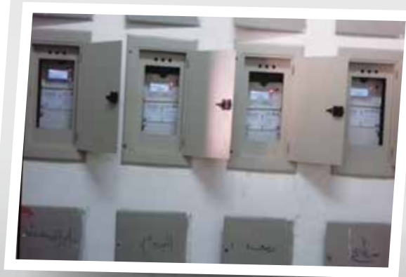
Installed Smart-meters
