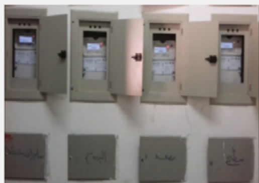
Installed Smart-meters
